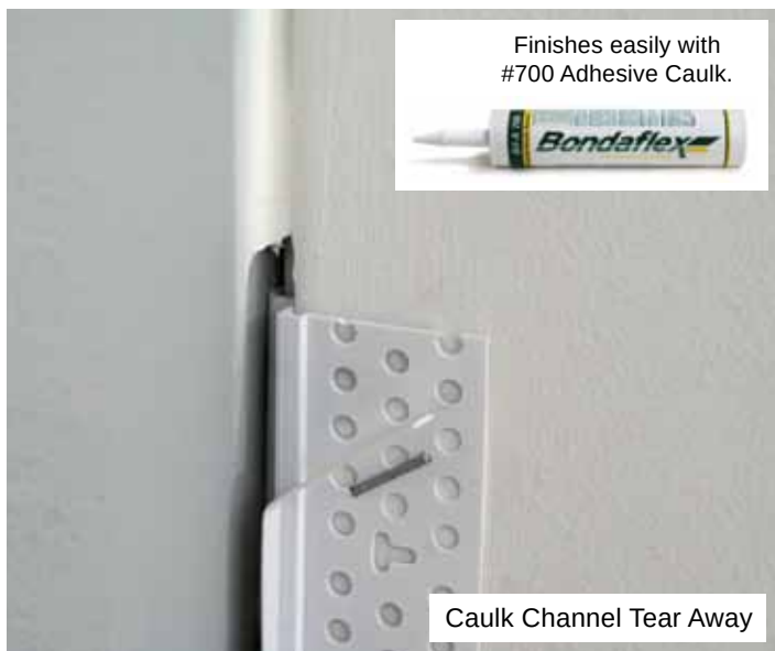
Caulk Channel Tear Away Bead Installation
