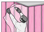
Applying vapour barrier
