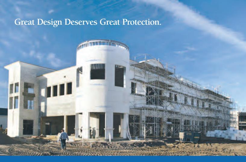
GlasRoc® Sheathing featuring patented\* Embedded Glass Reinforced Gypsum™ technology is strong, yet flexible enough to bend to curved surfaces like the towers at The Avenue at Westchase. Project: The Avenue at Westchase
